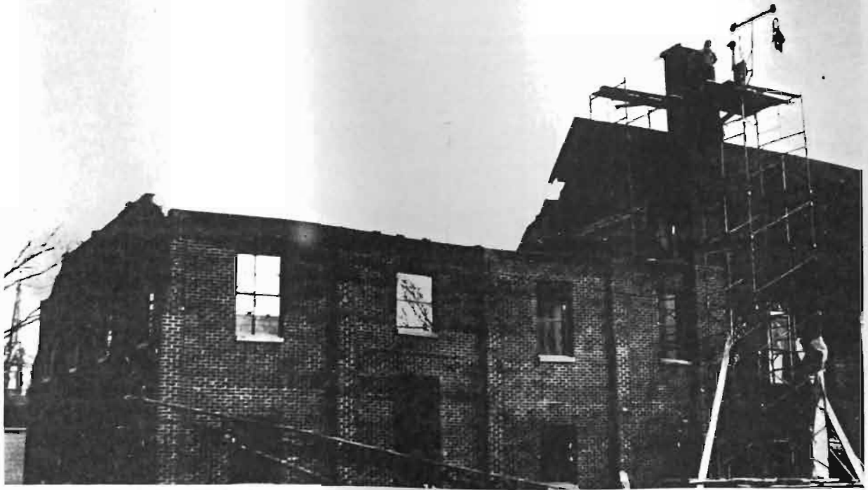
CHURCH UNDER CONSTRUCTION
