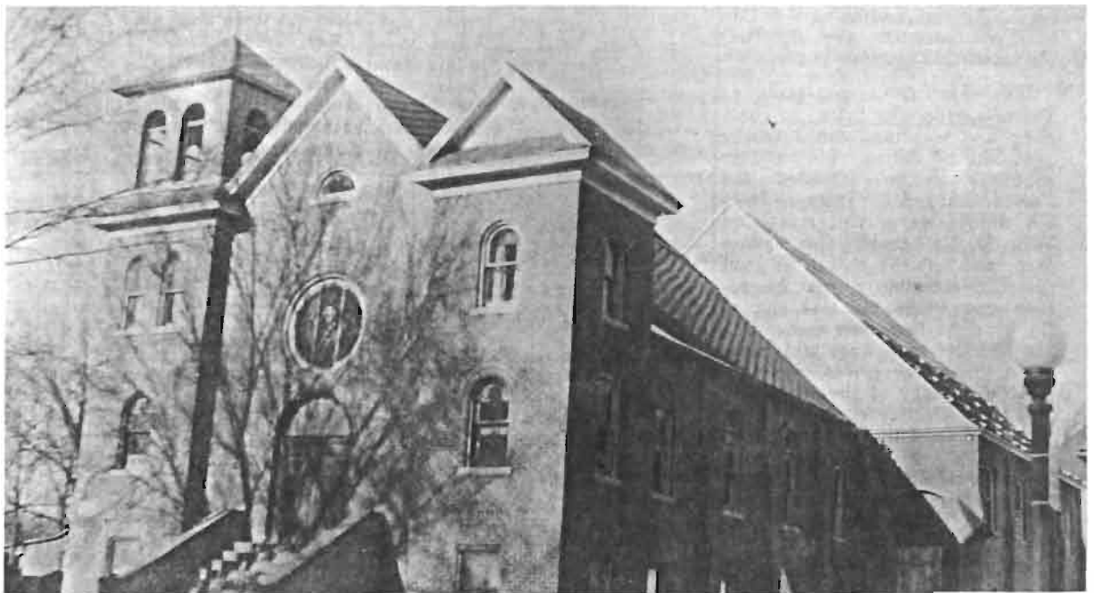
THE OLD FRONT PARK STREET
