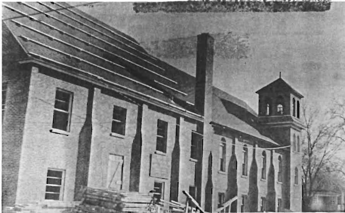
NEW ROOF - NO WINDOWS WEST SIDE LOOKING SOUTH
