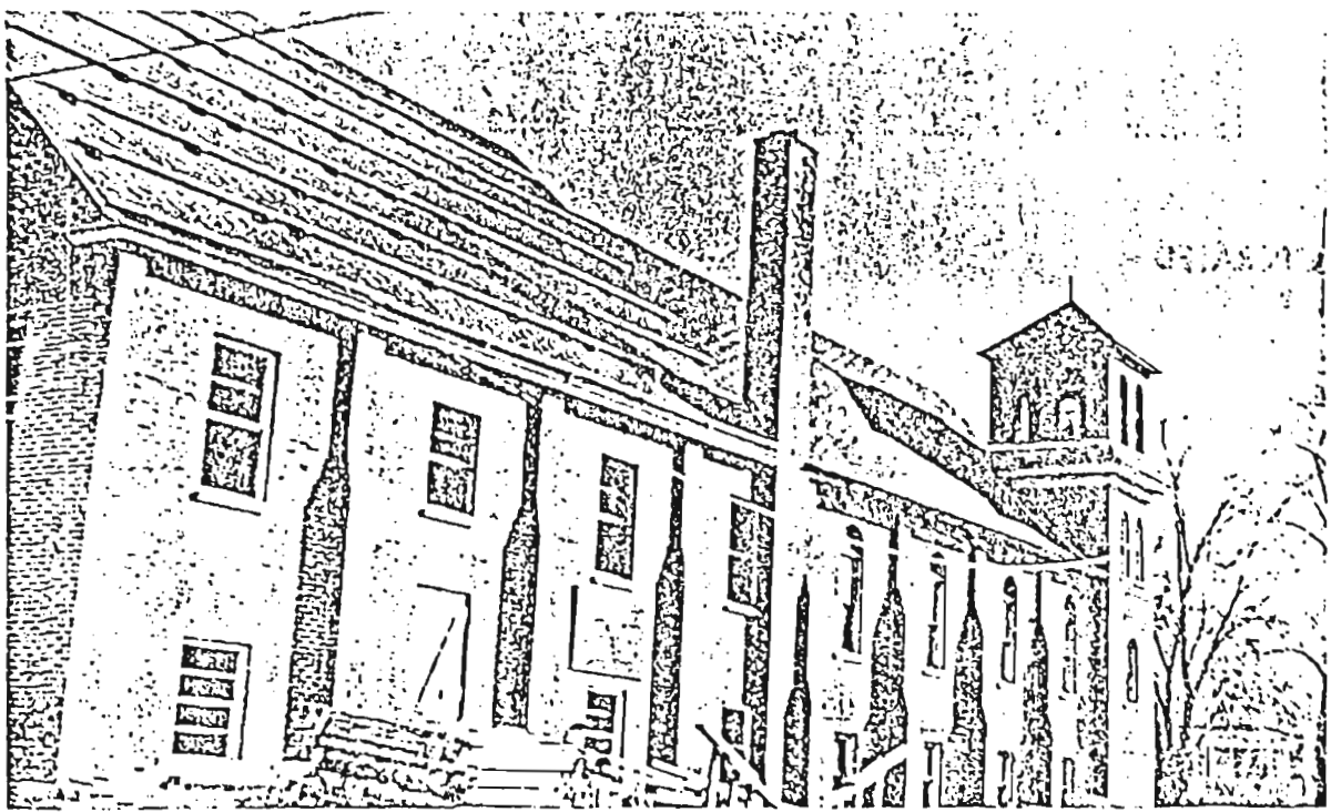
NO WINDOWS WEST SIDE LOOKING SOUTH
