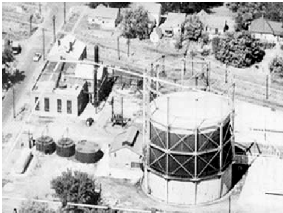
Fifth and Hill Site before removal of gas manufacturing plant in the 1950s.
