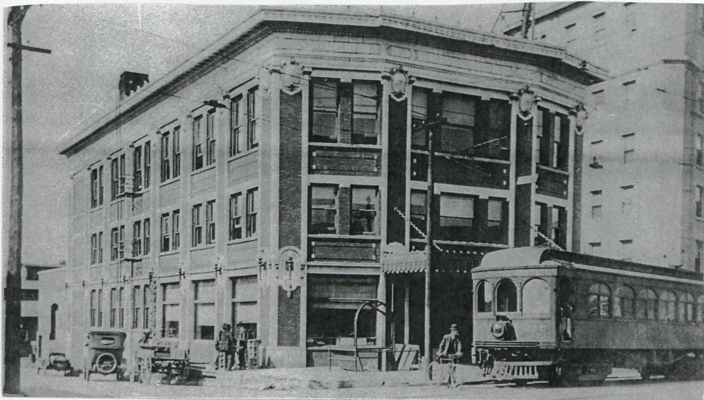
The station built by the Illinois Terminal in downtown Champaign in 1912. It also served as the ITR's main office building.
