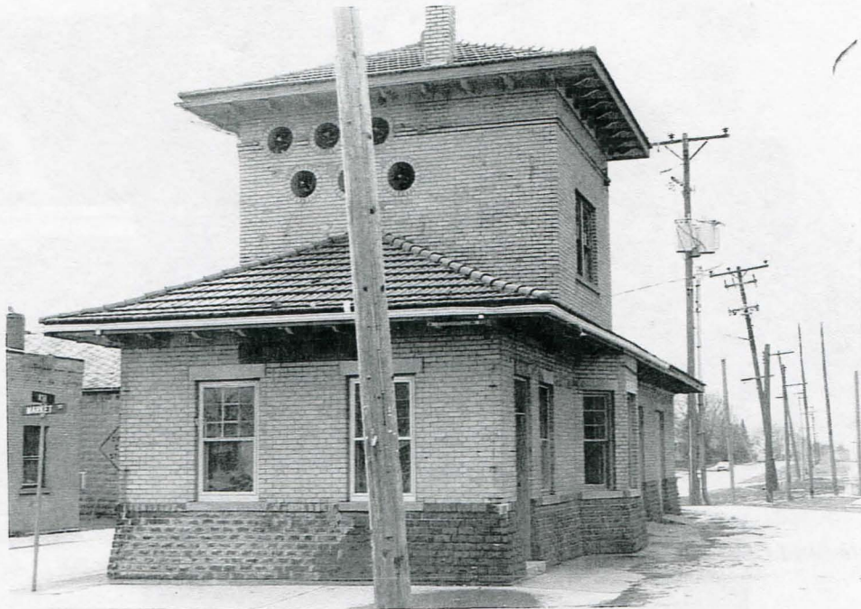
A view to the west of the former Illinois Terminal depot that still stands in Bondville. Power generators were in the depot's tower, and brick construction was used to minimize fire danger.
