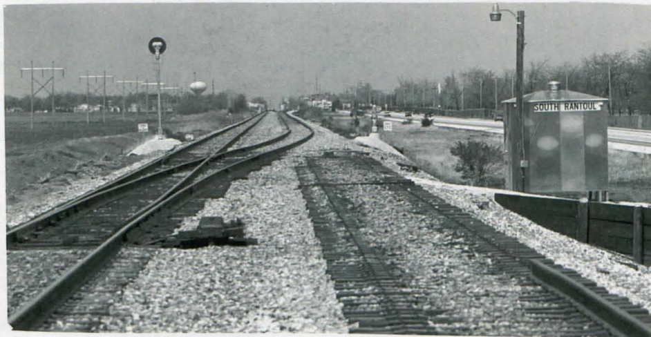
The IC's removal of its double track line is seen here near Rantoul in April 1990. Here, a portion of the once northbound line is being used as a passing siding. The removal of the rails and ties occurred 3 to 4 months later.
