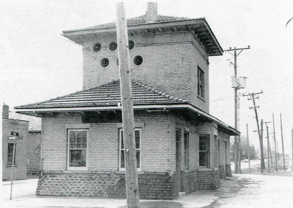
A view to the west of the former Illinois Terminal depot that still stands in Bondville. Power generators were in the depot's tower, and brick construction was used to minimize fire danger.
