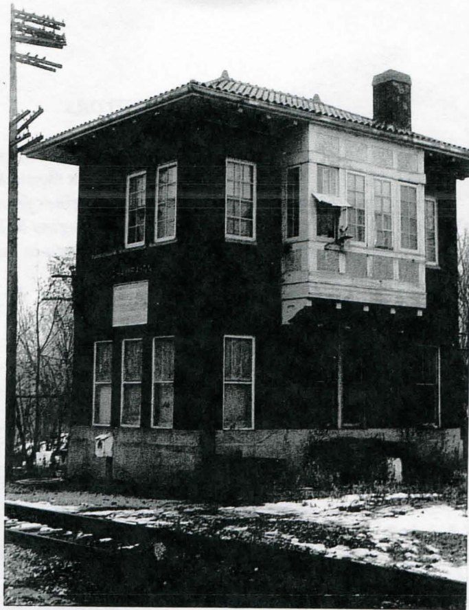
The brick control tower at the junction of the IC main line with the Conrail (former P&E) line in Champaign. The view is to the southeast. At one time, the Wabash line passed on the other side of the tower. The extended windows gave the operator a good view of the IC lines.
