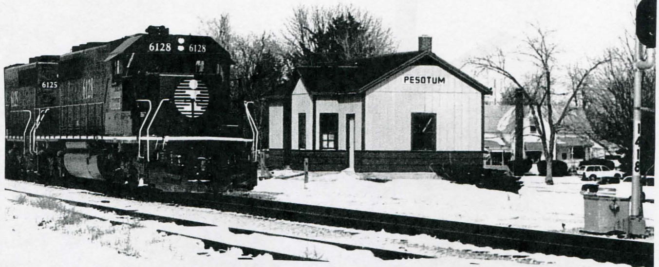
When the IC decided to tear down its many wooden depots in small Illinois towns, some persons and town leaders stepped forward and bought the stations. Here, the wooden depot at Pesotum, which has been restored and locally maintained, is passed by a southbound freight on a snowy December 1992.
