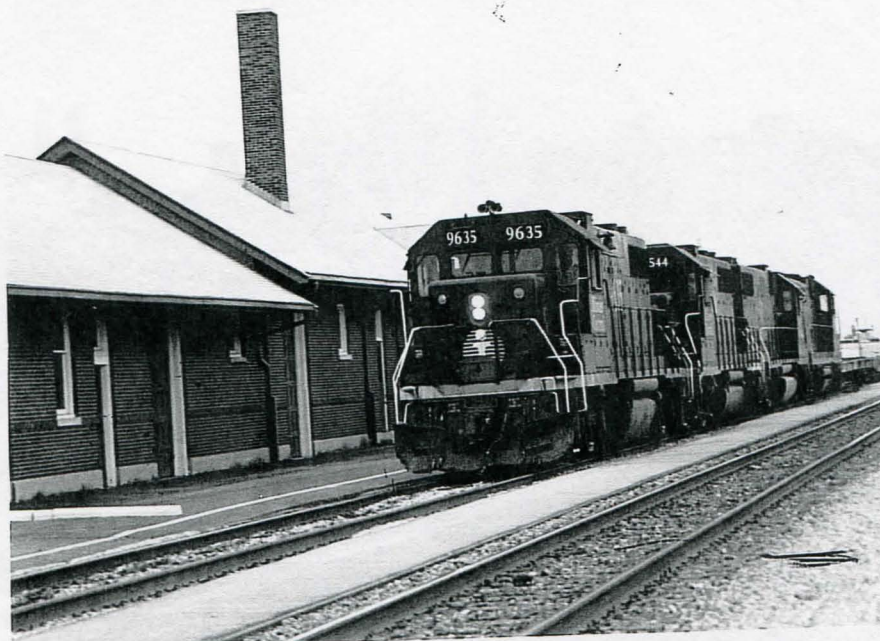
The former IC depot at Rantoul, now used by Amtrak, is being passed by a northbound IC freight.
