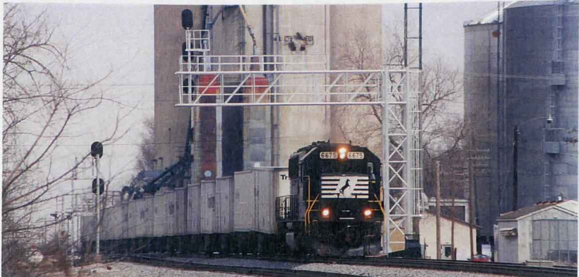
New signals were installed by NS at Tolono, reflecting their enhancement of control of added train traffic through town, as a westbound Roadrailer train passes beneath one of the new signal bridges.
