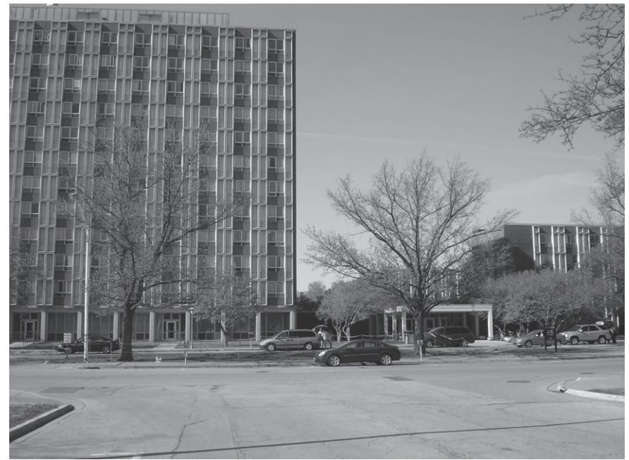
Illinois Strees Residence Hall - Home of most "Project 500" students.
