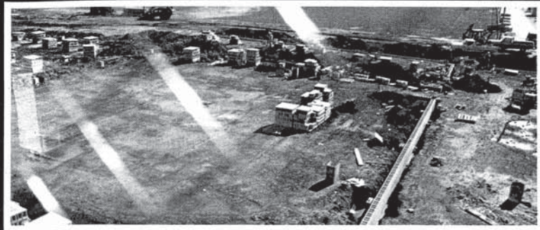
The future gym stands unfinished
