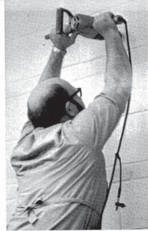
This is "bore-ing."
