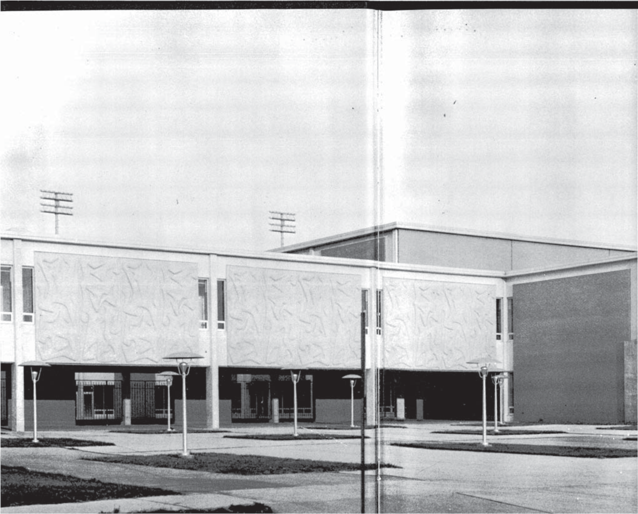
Out of a brush-covered field grew concrete walls, surrounded everywhere by a conflict of
