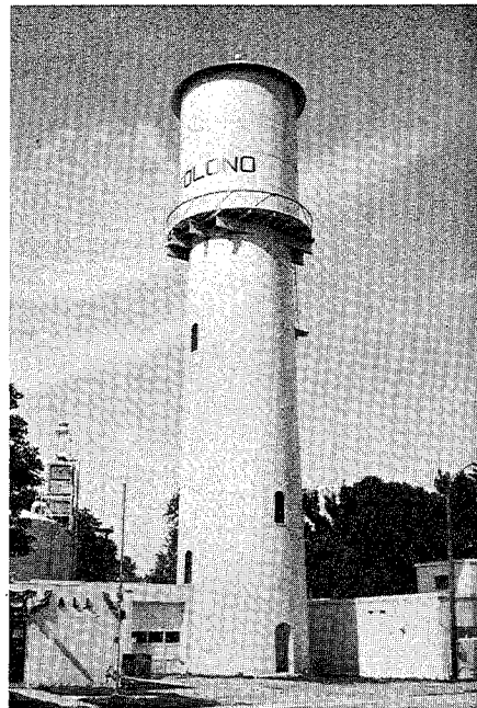
Tolono Water Tower
