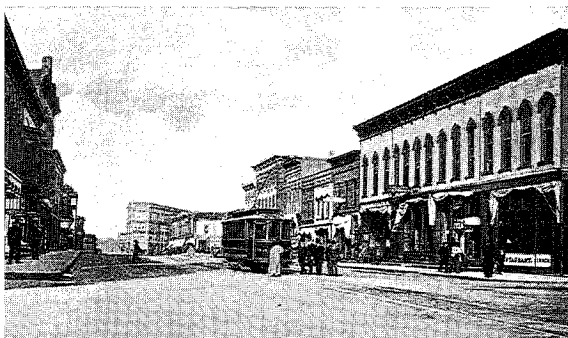
Looking West on Urbana's Main Street
