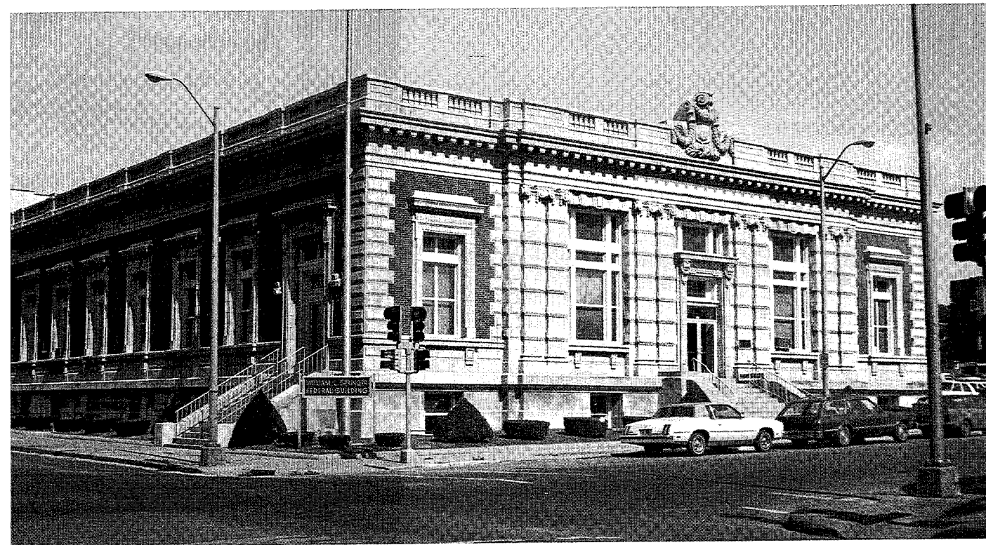
William L. Springer Federal Building Northwest Corner, Randolph and Church Streets, Champaign
