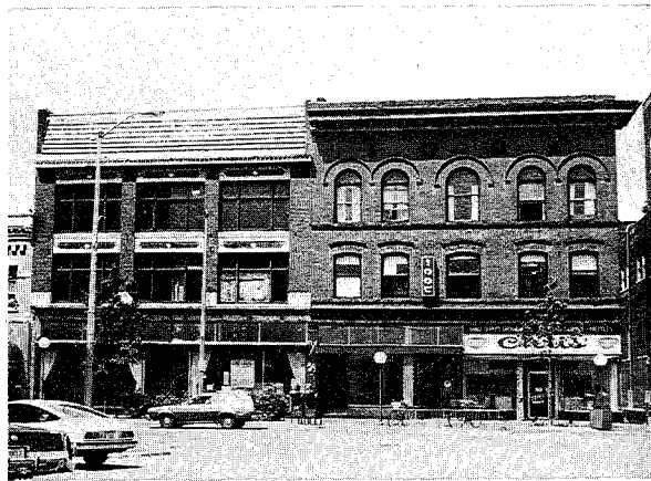
101-111 North Neil Street, Champaign (Demolished, 1981)
