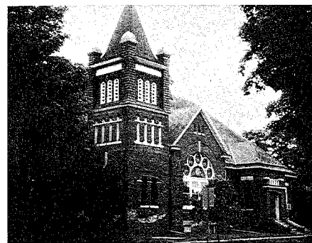
Old Sidney Methodist Church, Main Street The building is now a private residence.
