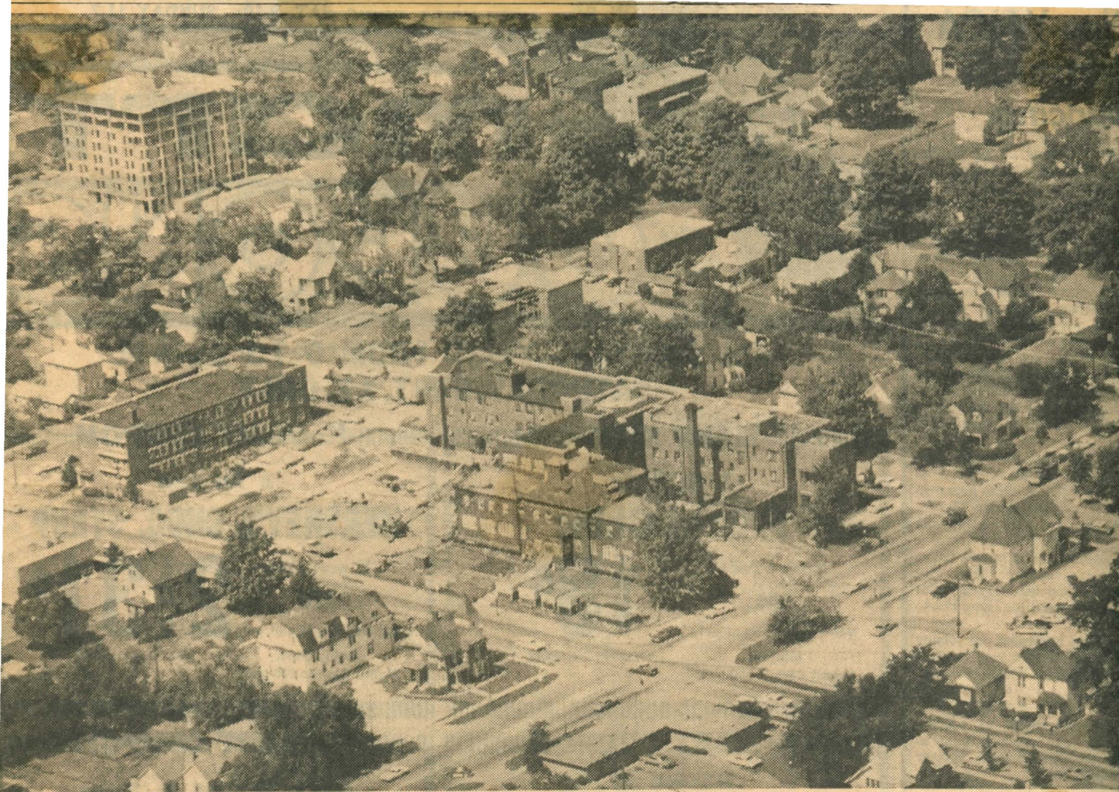
CH, PUBLIC HOUSING PROGRESS. Construction of the more than $5 million expansion of Burnham City Hospital, in center of picture, is progressing on schedule, according to Charles Becker, administrator. The project is being done in three phases. Demolition of the building at the front on Springfield, built in 1895, is scheduled for
