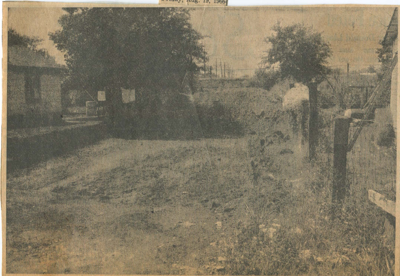
Foundation Hole at 803 N. Oak St. Awaits House Moved From 1st and Springfield
