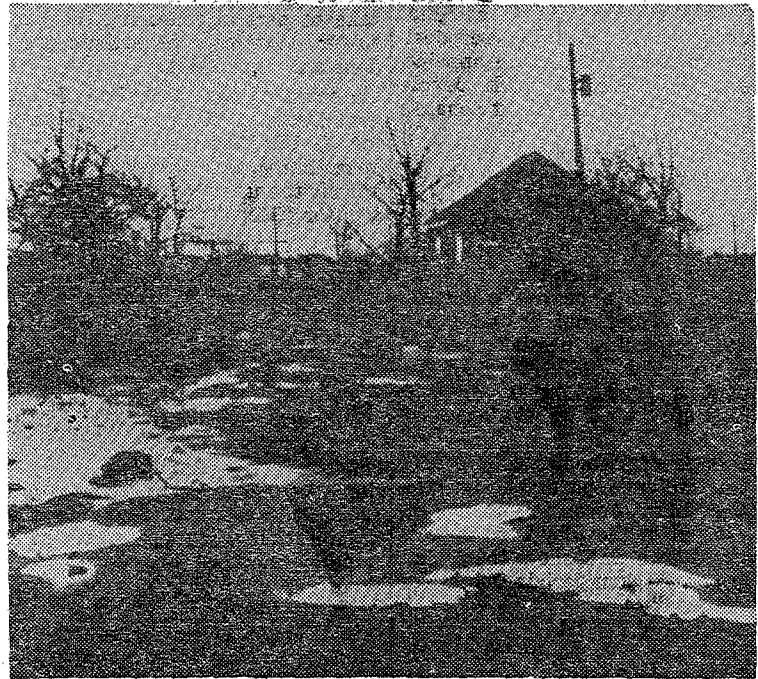
EMPTY LOTS PREDOMINATE in much of Champaign's largely black North End. Project of the city's urban renewal program has cleared some 66 acres of substandard housing. This land now awaits construction of replacement housing.
