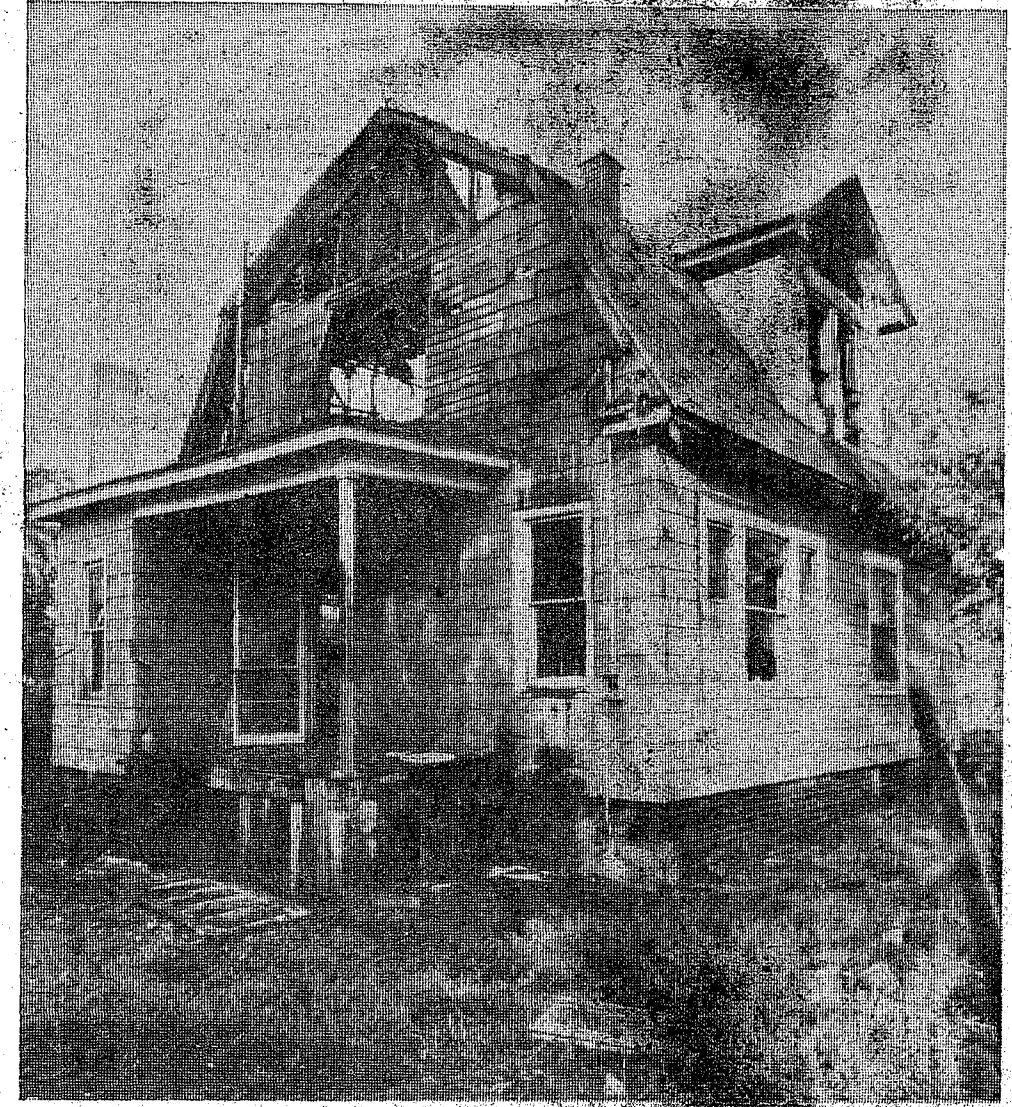
Rear of house extensively damaged by fire at 1106 N. 6th St.
