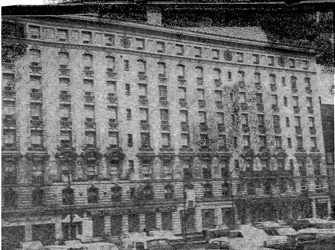
Brunswick Hotel is slated for demolition in redevelopment project.
