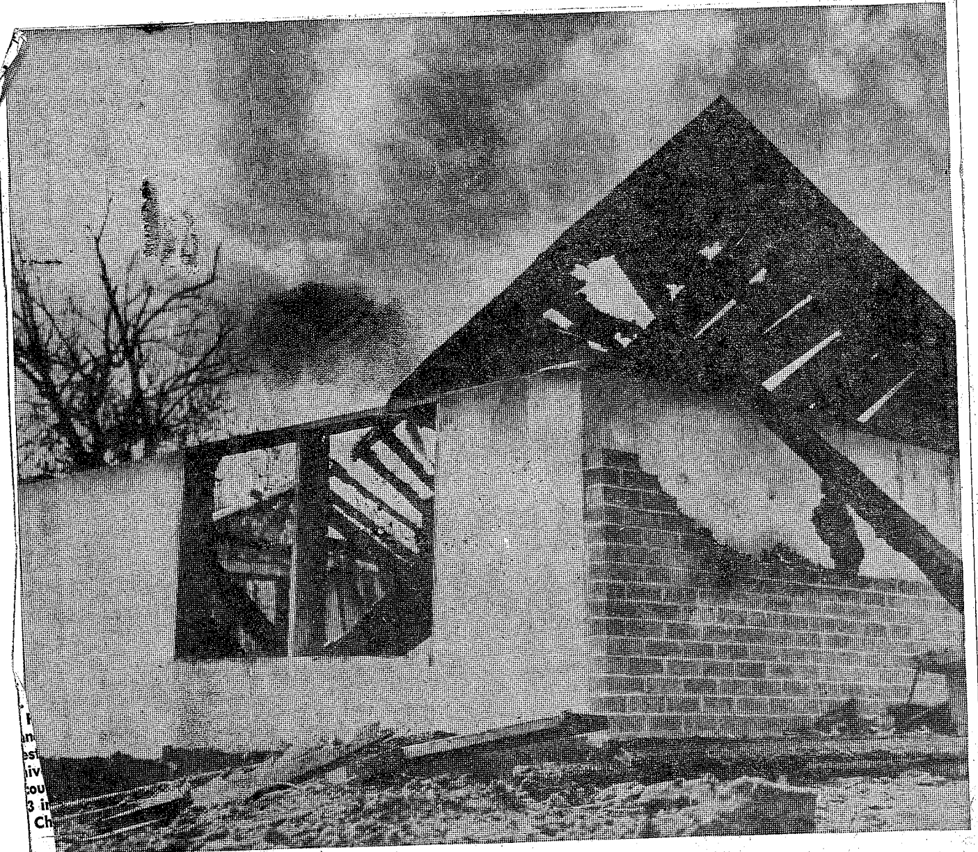
PARSONAGE RAZED re Thursday night de- ived Baptist Church, 1108 N. been completed; it was listed ect. Cause of the fire is not ed the partially complet- 6th St., Champaign. About half as a total loss by Action Real- yet known. ew parsonage for Mt. Of- of the $30,000 structure had ty, contractors for the proj- (Photo by Jim Rutledge)
