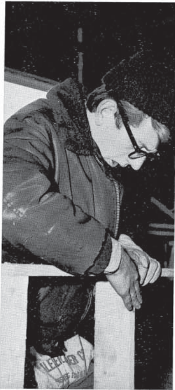
Bob Green braves a chilly fall morning to continue work on the Project House.
