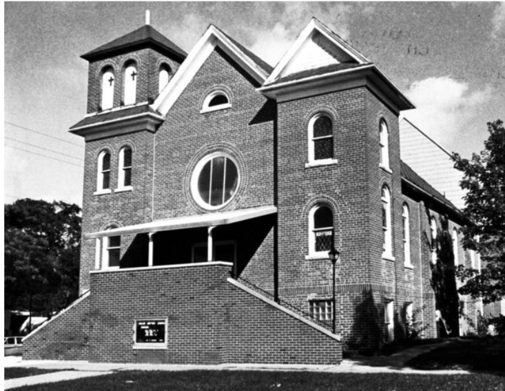
Figure 1. 500 East Park Street location prior to remodeling.
